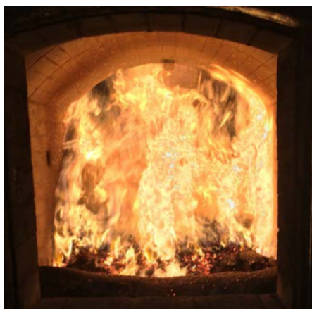
KPR System 5 MW
